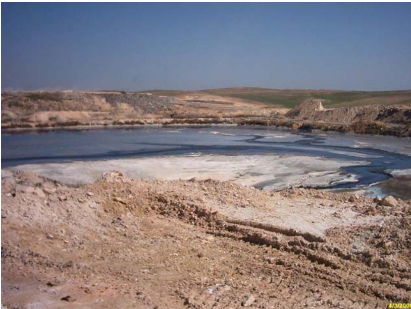
Figure 3: One of the lagoons where sludge is accumulated and left unmanaged in the foreground.
