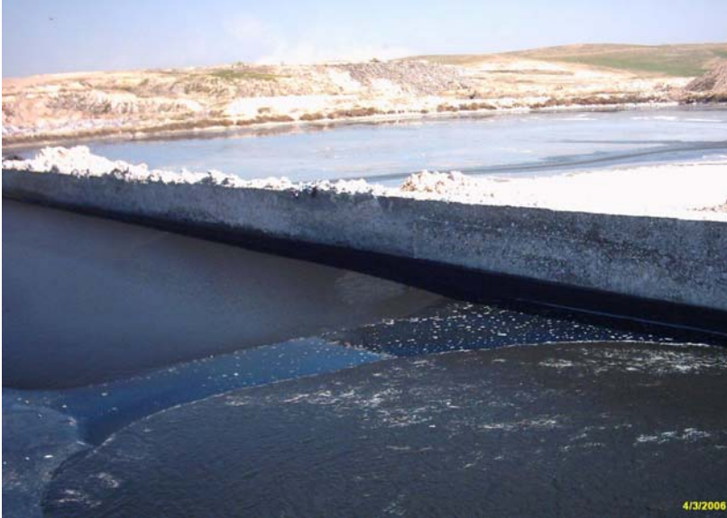
Figure 2: One of a series of waste lagoons showing what is known as blue wastewater in the ponds.
