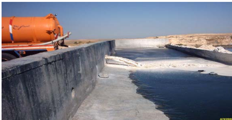
Figure 4: Tanker truck discharging waste to the distributor head
